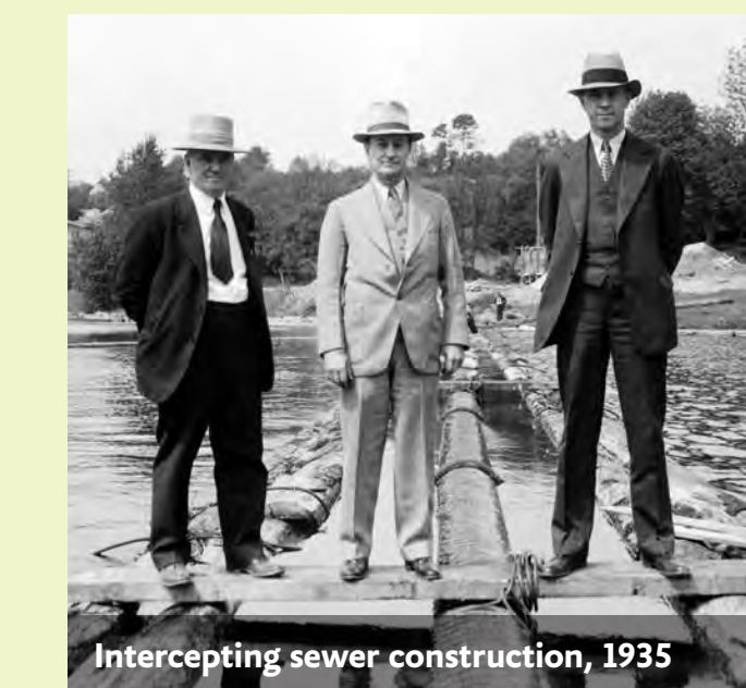
Intercepting sewer construction, 1935
